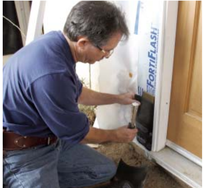
Figure 3. Covering the 1/2-inch plywood spacer with building paper (above) helps prevent water from moving between the wood trim and the plywood block. All cut edges should be primed before installation (left). Note the 1/2-inch jamb extension (below), which brings the back of the trim out flush with the top of the spacer blocks.
